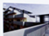
From above, the building's unique residential units would be a perfect fit for the type of work that OPEN likes to do in Shanghai, based on a recent precedent. OPEN had been a major model, but it seems the firm was not interested in the form there in its
