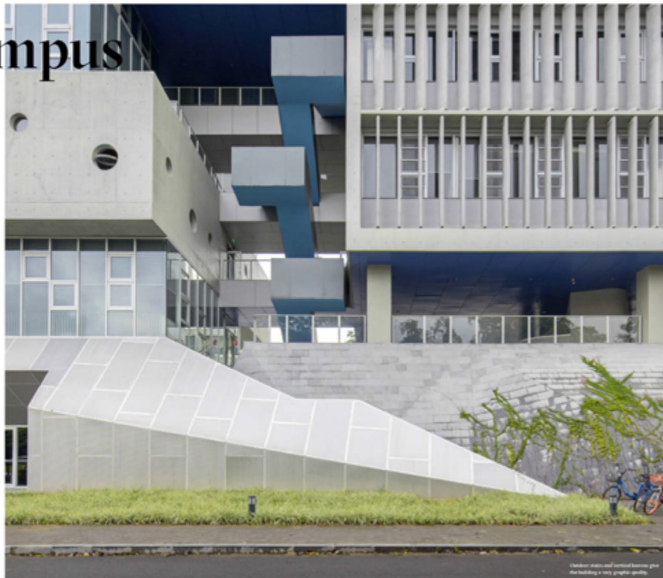
Outdoor stairs and vertical louvers give the building a very graphic quality.
